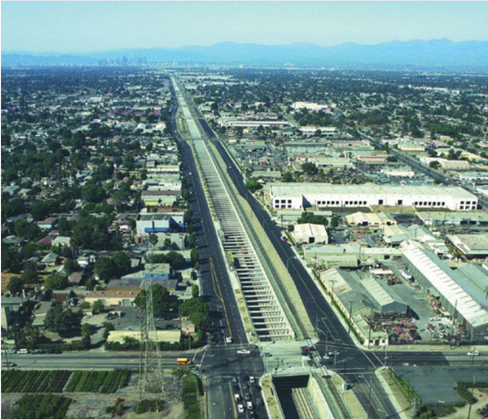
The Alameda Corridor Project built a rail access network to the ports of Long Beach and Los Angeles.
